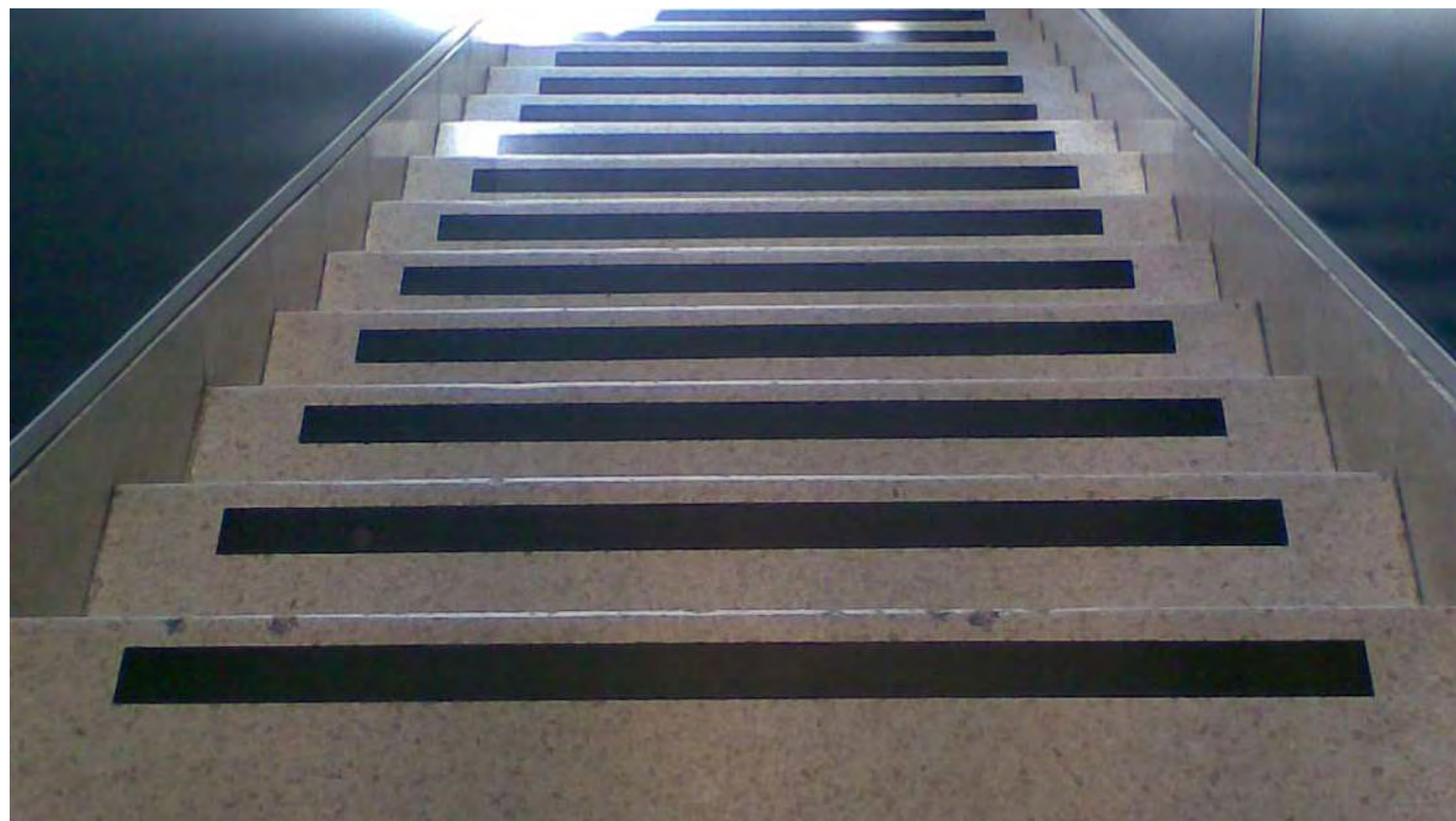
POOR POSITION – Does not define step nose
