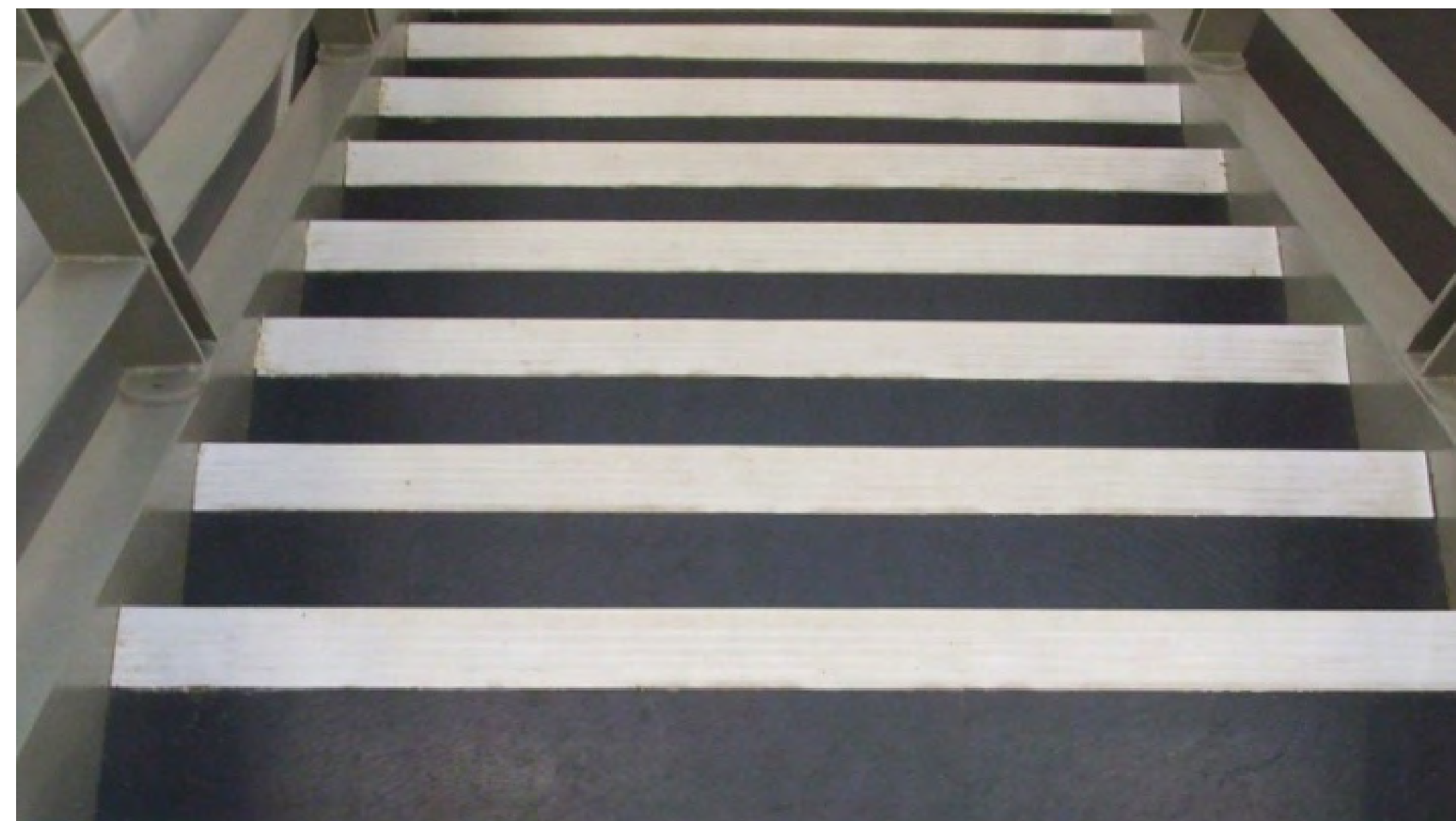
GOOD POSITION – Clearly defines step nose
